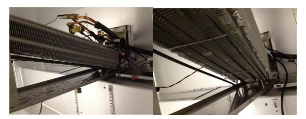
5. Unplug defrost heater connections and fish out of housing, angle front side upwards as much as possible and remove the either side of the housing. Once removed test resistance again. If determined the defrost heater needs to be replaced. Check with your supervisor about returning the defective part to Traulsen.
