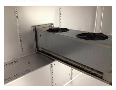
**3.** Next remove the dual evaporator fan panel on top, followed by the two galvanized side pieces. A few zip ties may need to be removed to allow slack to set this piece aside. This would be a good point to test the heaters resistance before proceeding any further.
