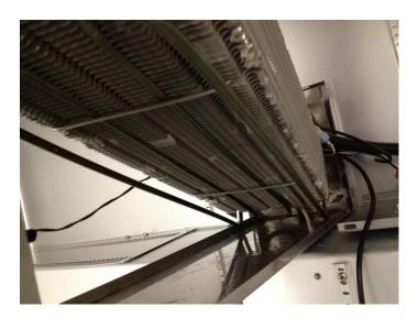
7. Lower evaporator back into position and secure with screws removed earlier.
